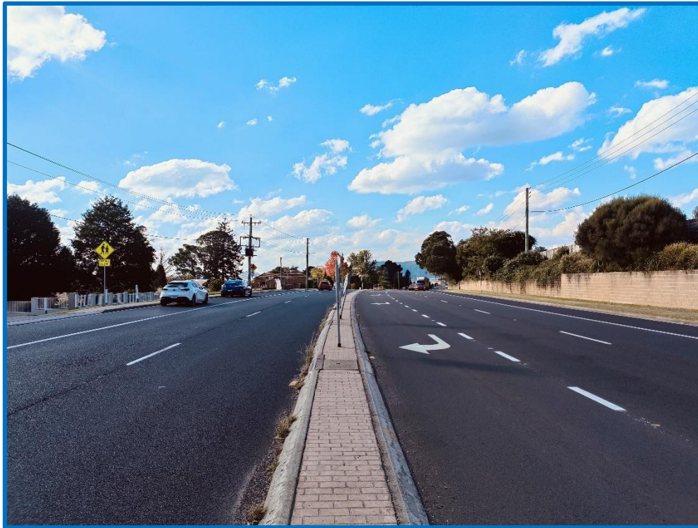
Figure 4b: Great Western Highway looking North from the intersection with Magpie Hollow Road
